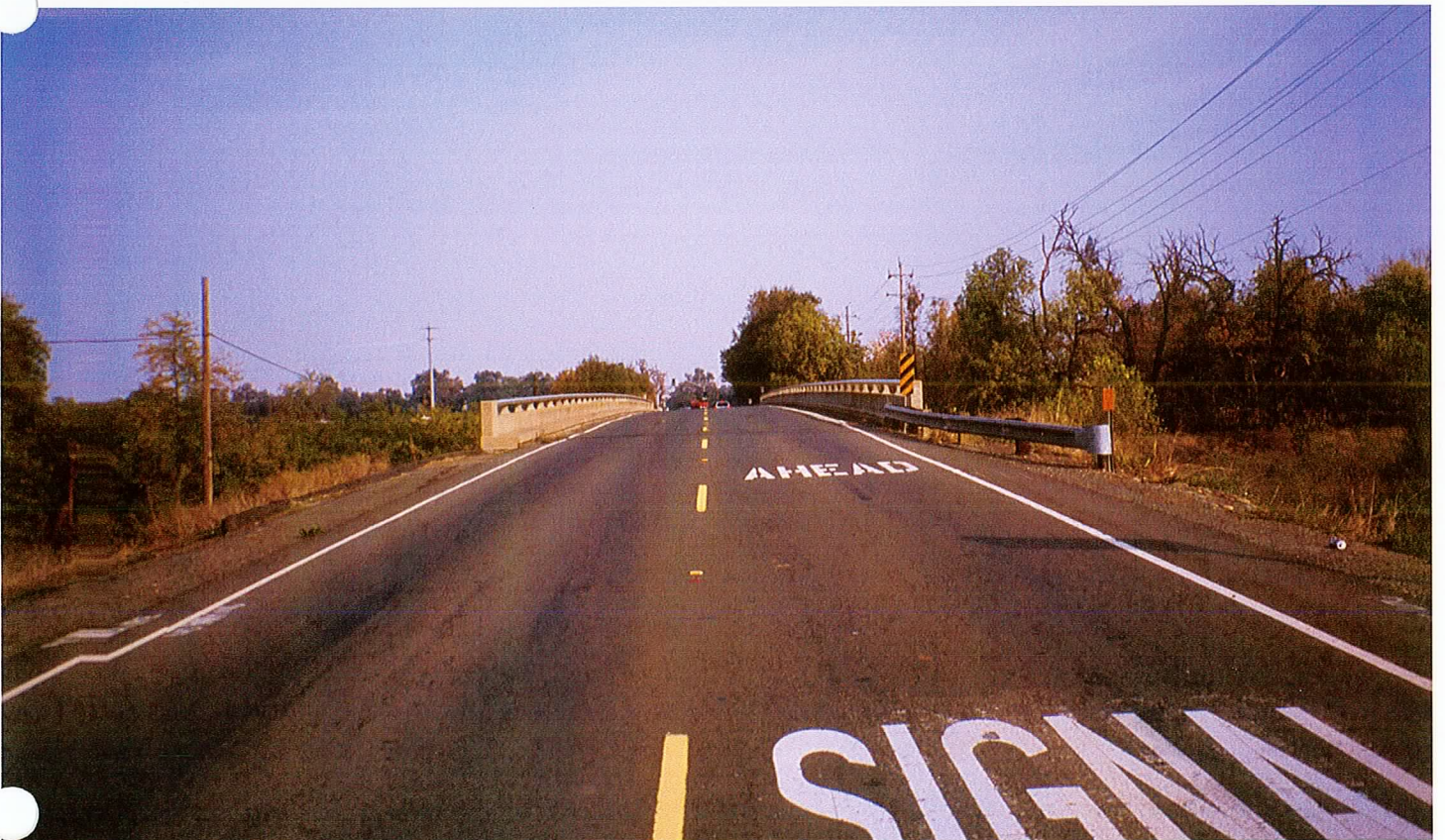
ROADWAY: Looking North 03-Sac-Co.Rd., Br#24C0004, Cosumnes River, 11-15-01, 06B-Sac2-20
