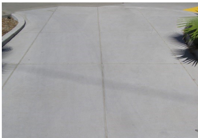
Score-Lines are a Simple and Cost Effective Enhancement of Standard Sidewalks
