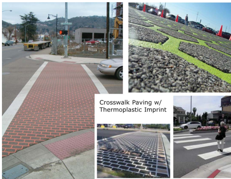
Examples of Crosswalk Paving with Thermoplastic Imprint
