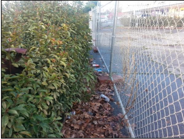
Improperly installed fencing allows access onto private site. January 2016.
