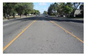
Existing Condition: Four lane roadway with a two way left turn lane and no bike lanes.
