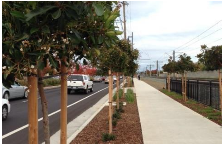
Bifurcated sidewalk construction along Folsom Boulevard within Rancho Cordova
