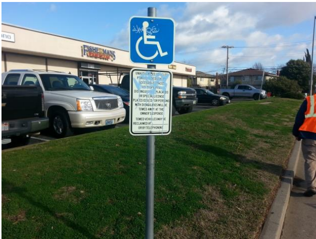
Existing signs are regularly vandalized
