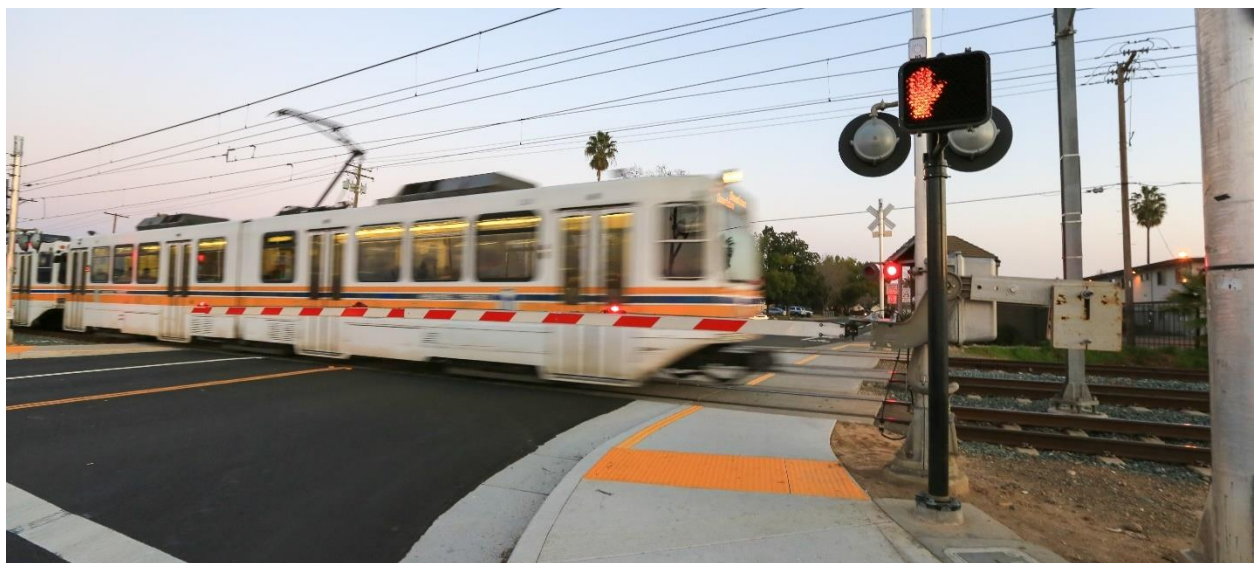
The Sacramento Regional Transit Gold Line runs parallel to Folsom Boulevard and creates opportunities for transit riders but also has challenges for automobiles at the various at-grade crossings.
