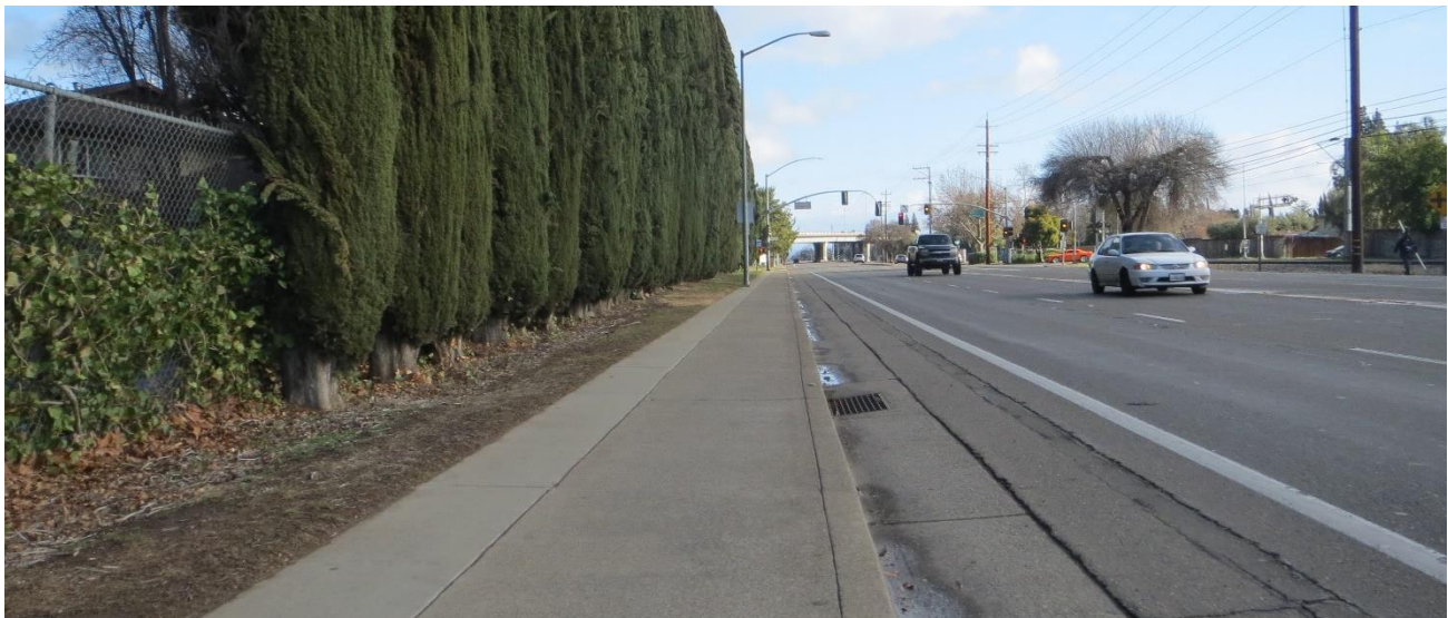
Attached sidewalks and and minum width Class II bike lanes that exists on portions of the boulevard can be enhanced to promote more active transprotation uses.
