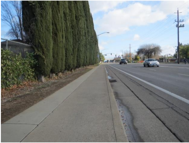
Vegetation can obstruct line of sight as easily as a solid wall.
