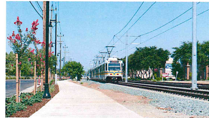
DETACHED WALK (RAIL SIDE)
