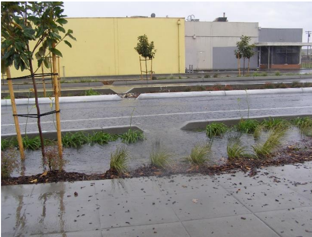
Example of a storm water retention at Freedom Park Drive in Sacramento County
